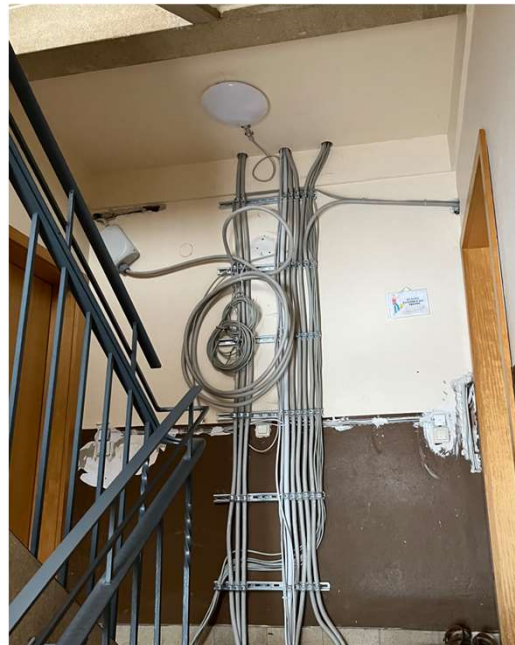
Rheinlandstr. 2-4 Neuinstallation Elektrik
